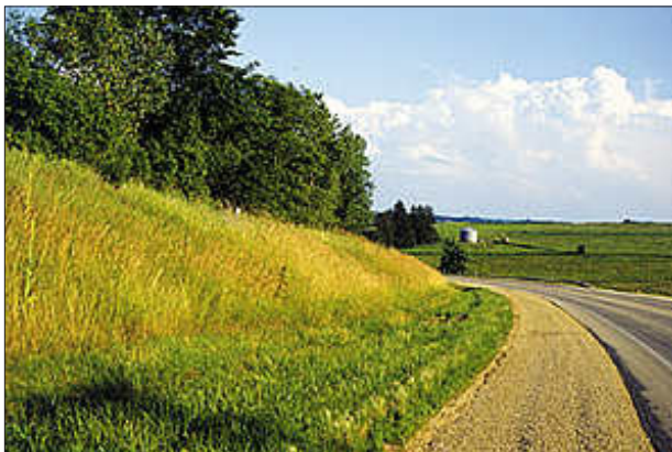
Landscape treatments along edges and medians that add visual interest and minimize on-going maintenance costs
