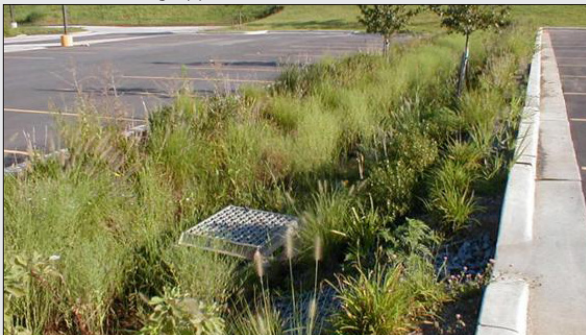
Raingarden to treat parking lot runoff
