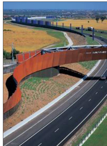
A pedestrian bridge crossing over an interstate that also serves as a piece of art
